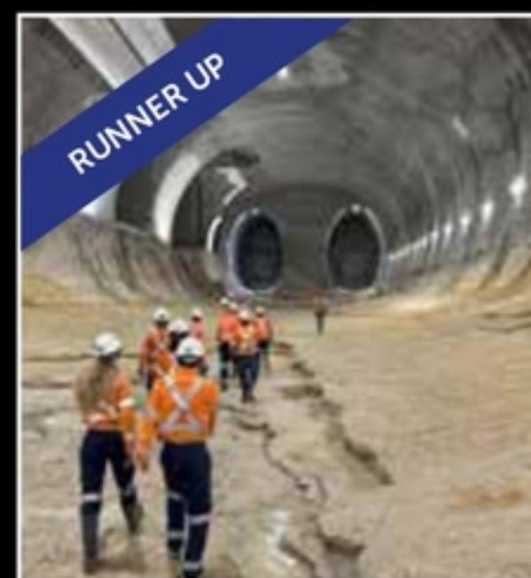
**Description:** These visitors are fortunate to see the Hunter St Station cavern at its most impressive stage, before the massive space gets progressively smaller with the construction of the permanent concrete lining and architectural linings.
