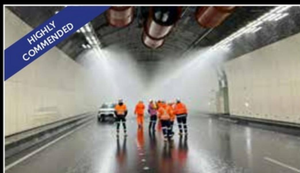
**Description:** Australia's first Tunnel Misting System in Operation at the recently refurbished Heysen Tunnels in Adelaide, South Australia
