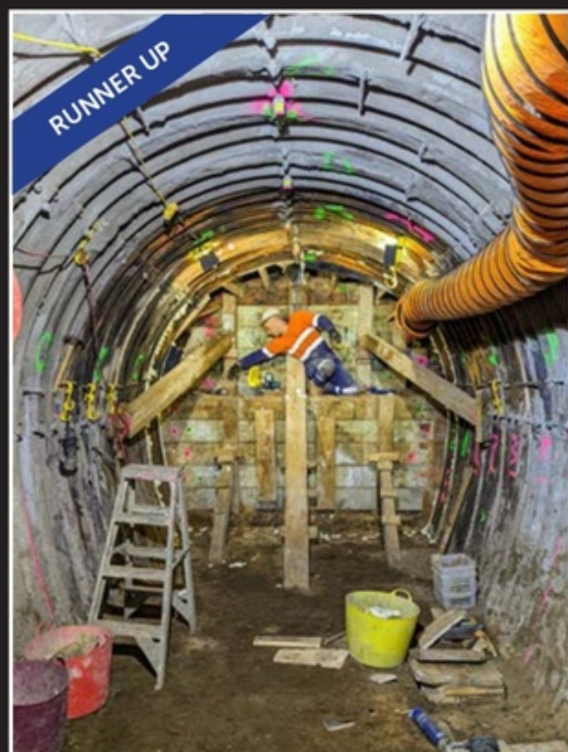
Sydney Wine Cellar Construction, by Quinn Kenny
