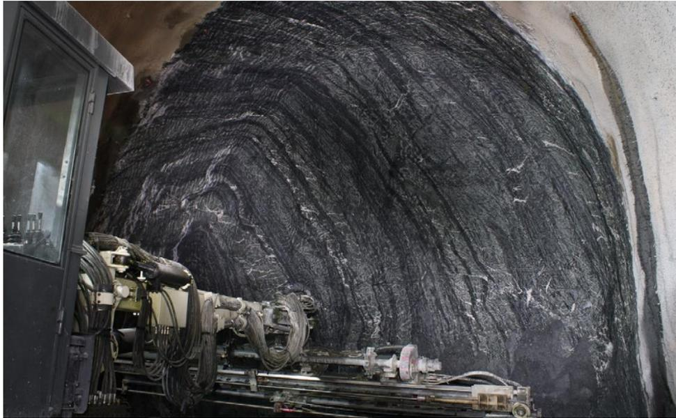
Figure 3. Typical fresh to slightly weathered NFG at Albert Street station from Cammack et. al (2022)
