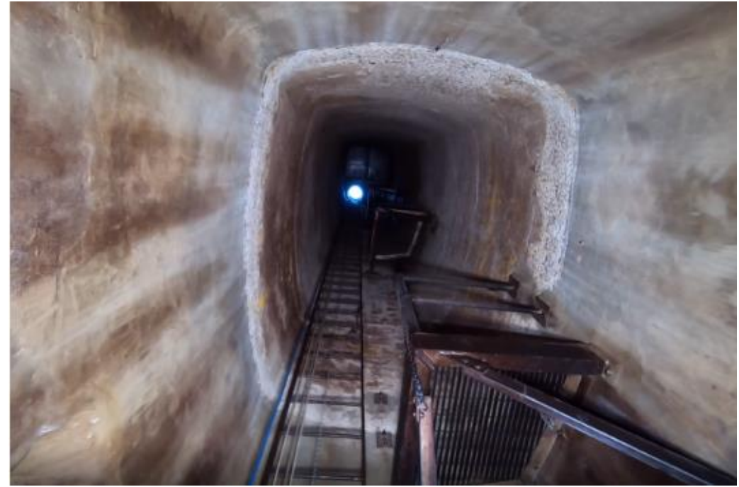
Base of manhole access
