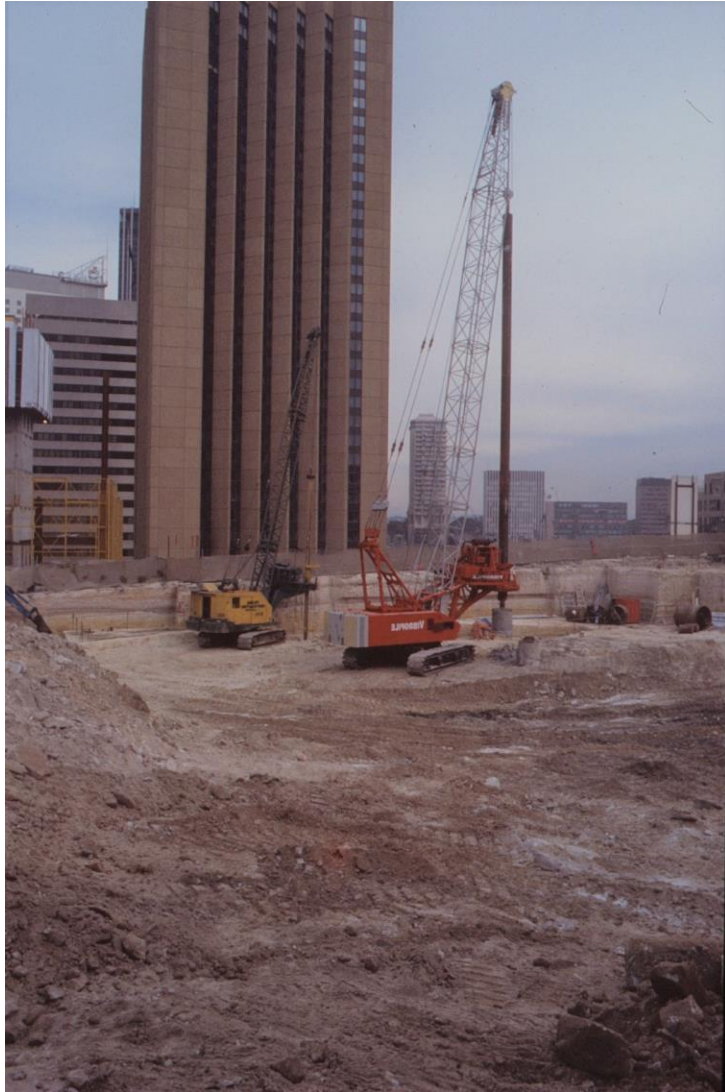
Piling – Shangri La Hotel – The Rocks - 1988
