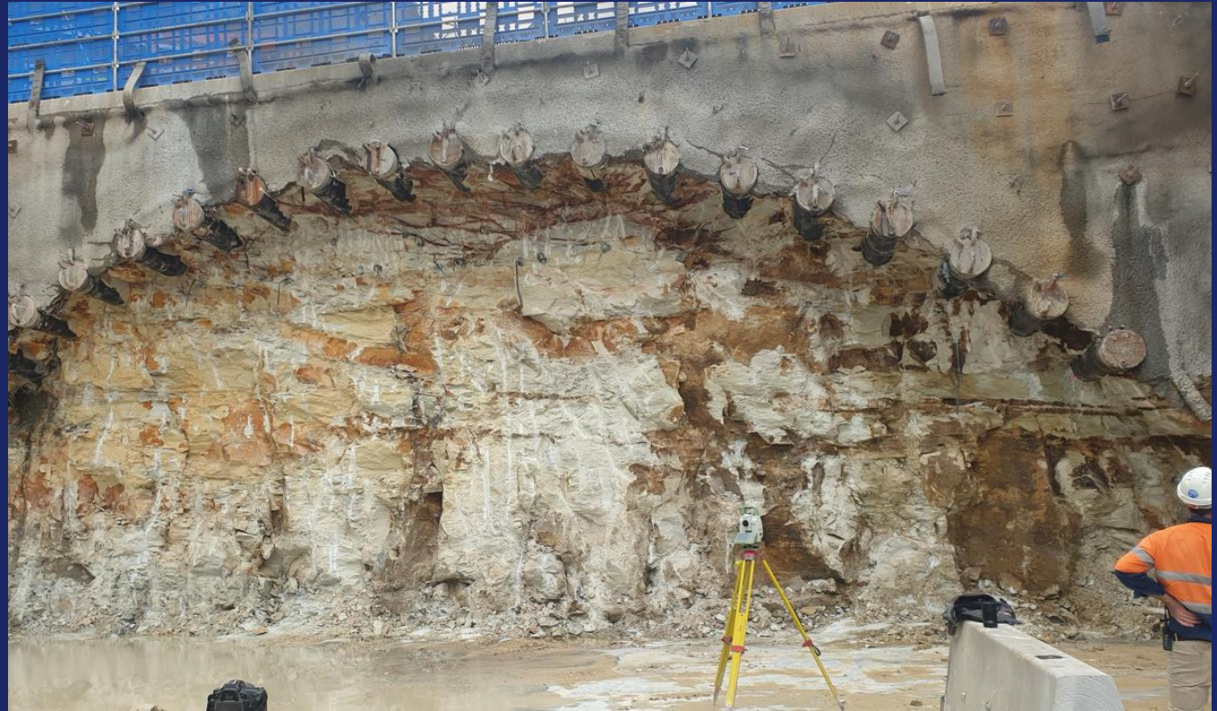
WEATHERED TUFF (BOGGO ROAD CAVERN)
