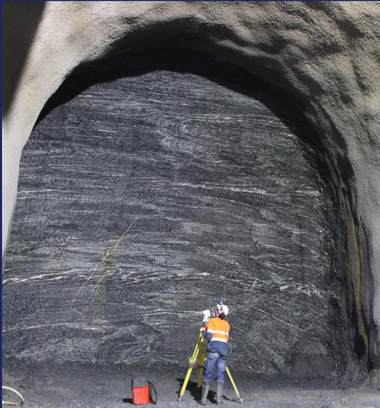
HIGH STRENGTH NERANLEIGH- FERNVALE GROUP (ALBERT STREET ACCESS ADIT)
