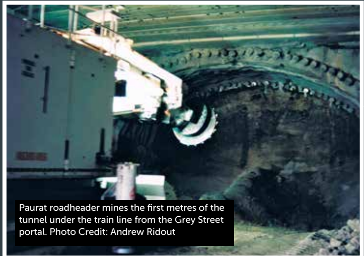
Excavation of the top heading under the already installed canopy tubes, steel sets and sprayed concrete. Photo Credit: Andrew Ridout
