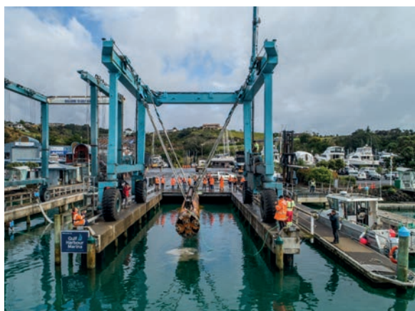
Retrieval of the MTBM at the Army Bay Ocean Outfall project
