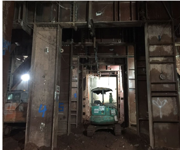
Fig 8. Site constraint for movement of excavators
