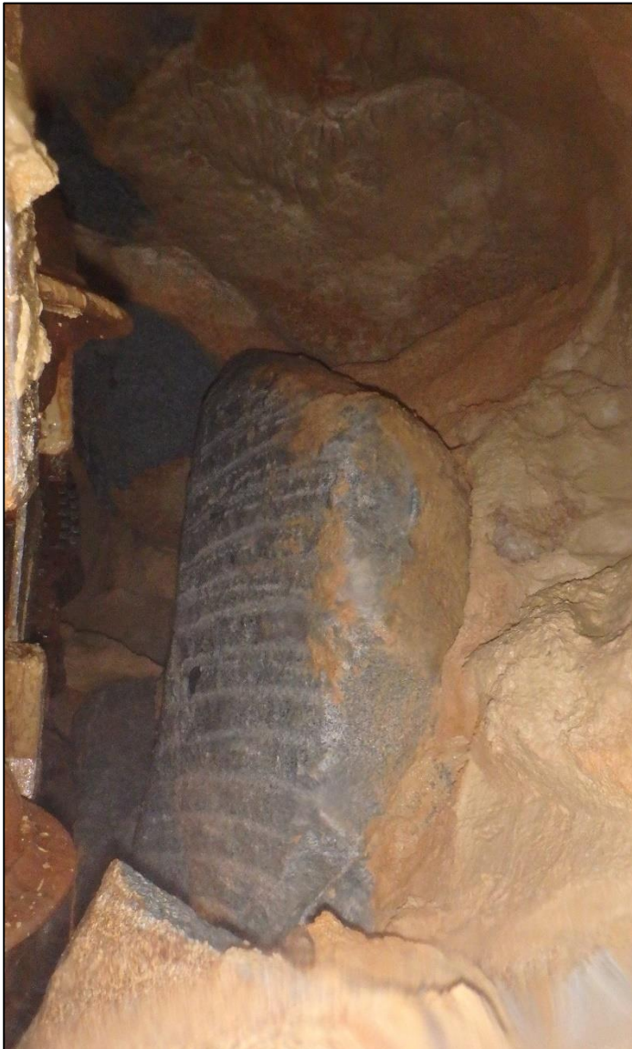
Figure 10: Large boulder encountered in front of the excavation face
