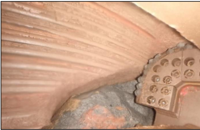
Figure 7: The application of a good bentonite face provides minimises slurry and air losses
