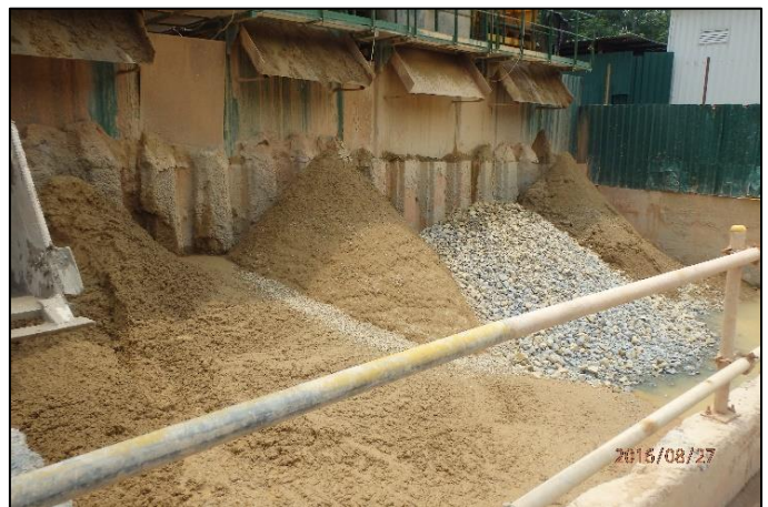
Figure 18: Manual volume checks at the STP in regular intervals supports the MRS. Any inconsistencies between the two systems can be determined
