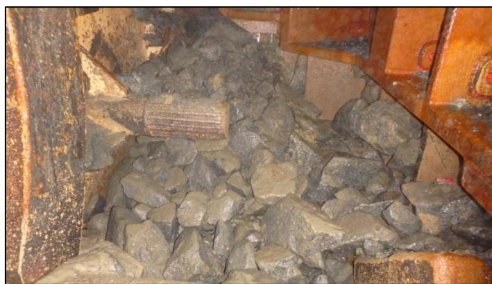
Figure 15: Blocked excavation chamber and bubble gate from smaller boulders
