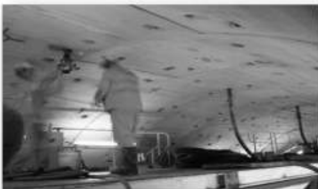
Figure 4: Secondary grouting of every second segment (courtesy Mr. Michael Huber) and potential insignificant primary grouting (modified from [11]).
