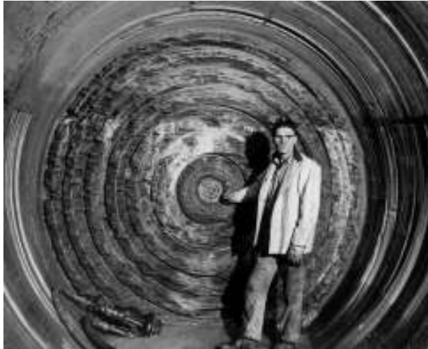
James S Robbins stands in front of an early TBM excavation face showing kerf cutting.
