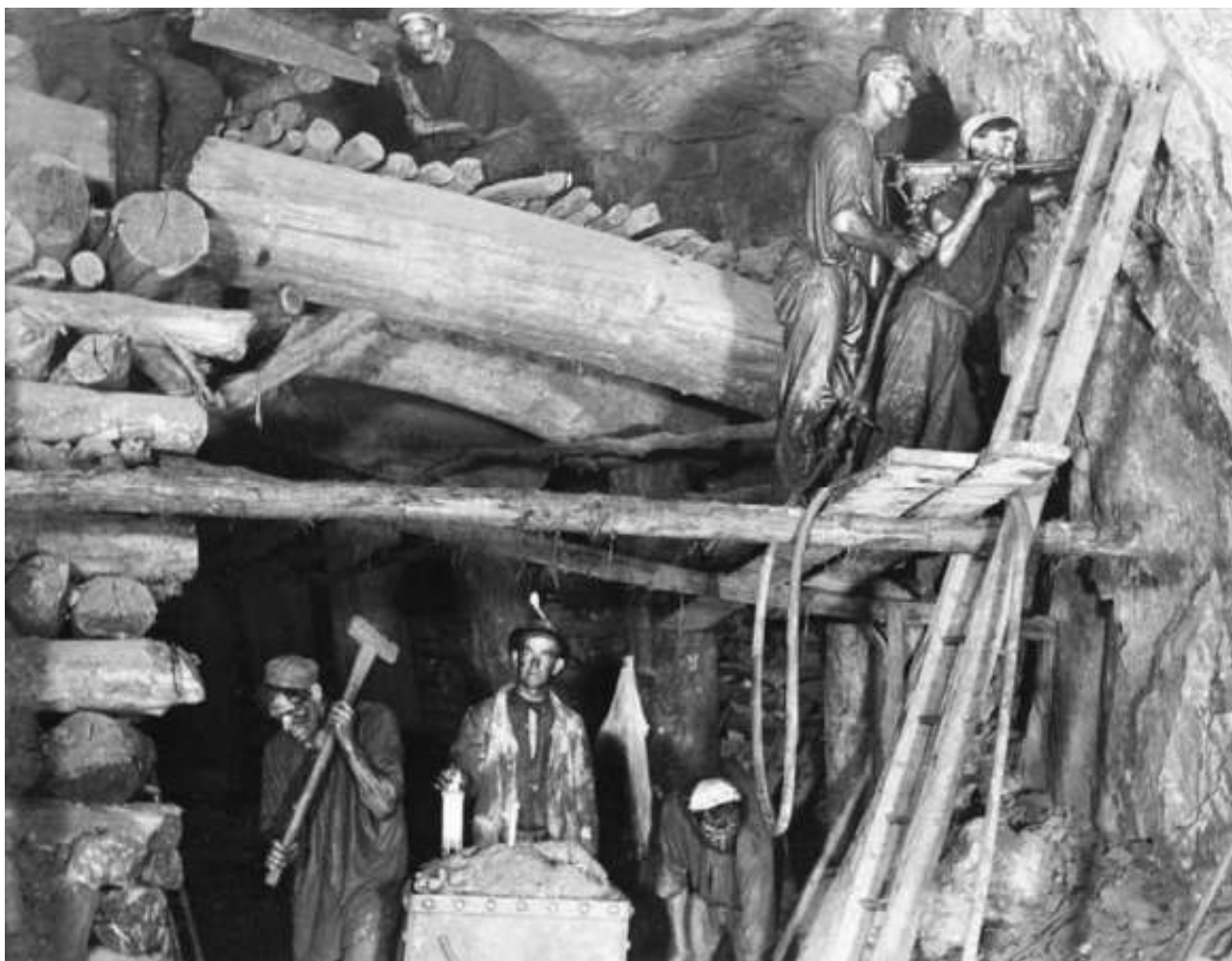
Overhand stoping at Wallaroo Mines, c.1915.
