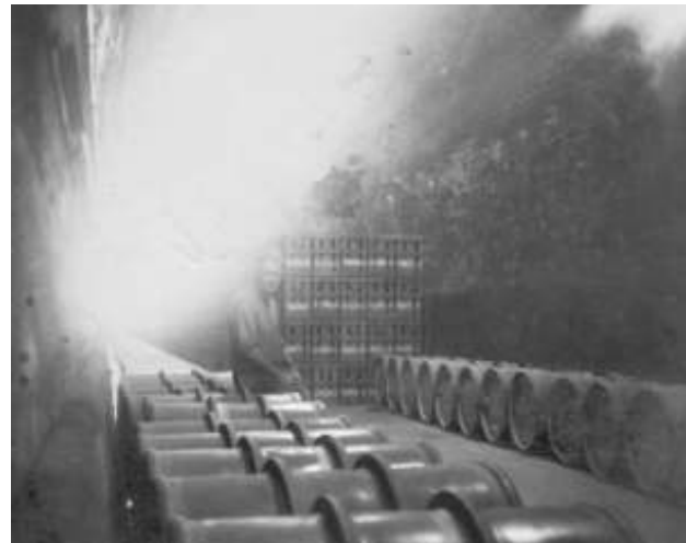
Chemical Special No. 6 mustard recharging drums inside the Glenbrook tunnel.
