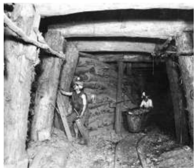
Loading from an ore stope in a well timbered drive, Wallaroo Mine c.1915.
