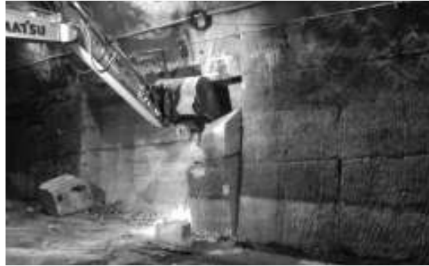
Hydraulic splitting work in the tunnel 25 June 2011
