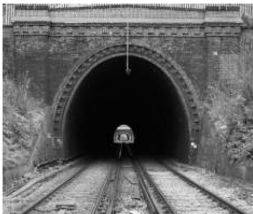
Charlton Lane tunnel
