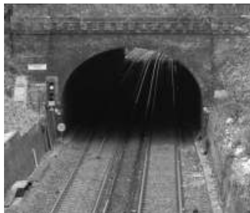
Mount Street tunnel
