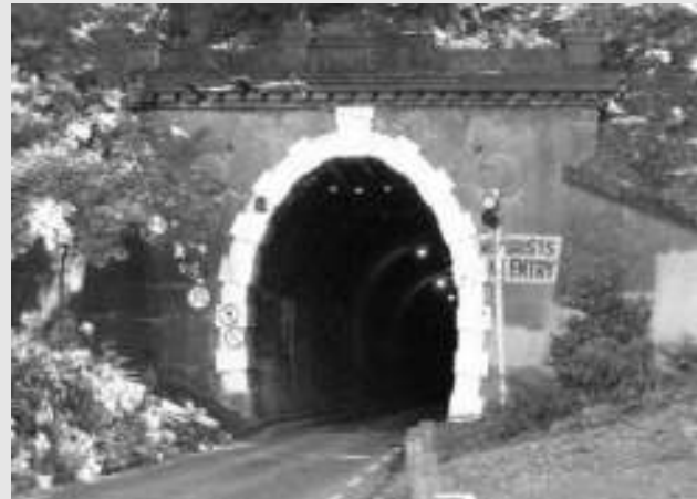
The Hataitai side of the tunnel at the end of Waitoa Road
