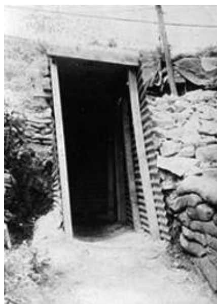
Sapper tasks included preparing shellproof fighting bunkers and machine gun posts with shellproof lintels.
