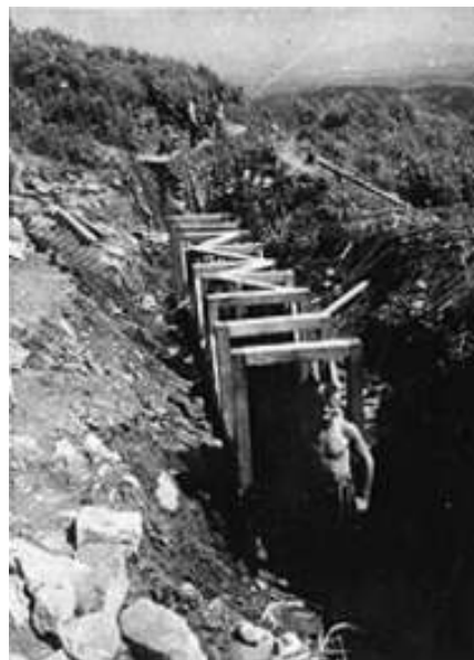
Cut and cover trenches were built with concrete lintels over observation posts (OPs) and medium machine gun (MMG) positions as an alternative to tunnels.
