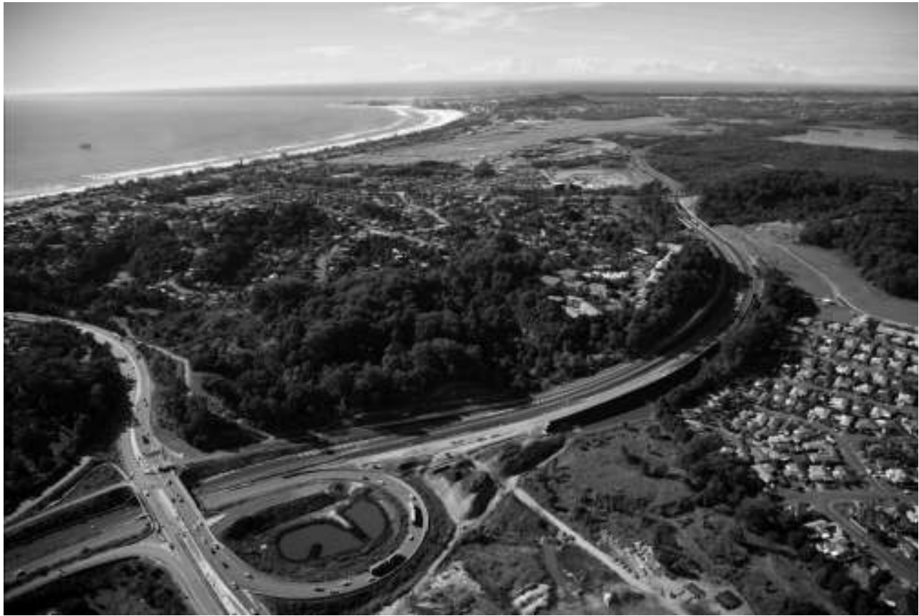
The Tugun Bypass viewed from the northern interchange at Currumbin, QLD
