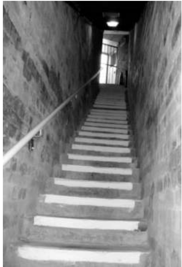
Stairs leading down to tunnels.
