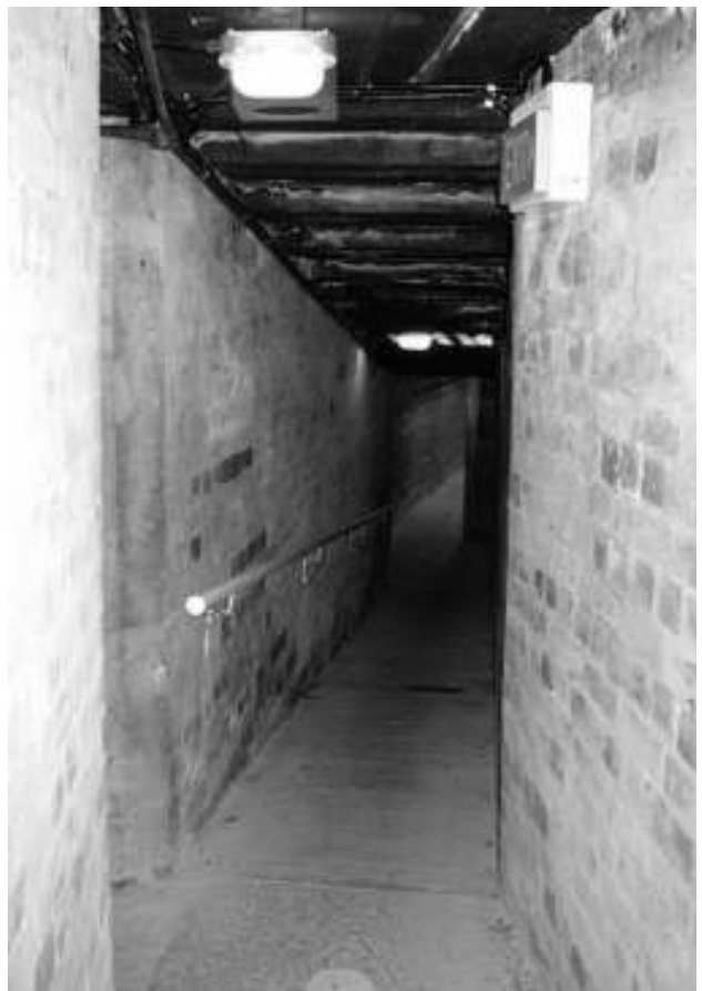
Underground brick lined corridor of Leighton Battery.
