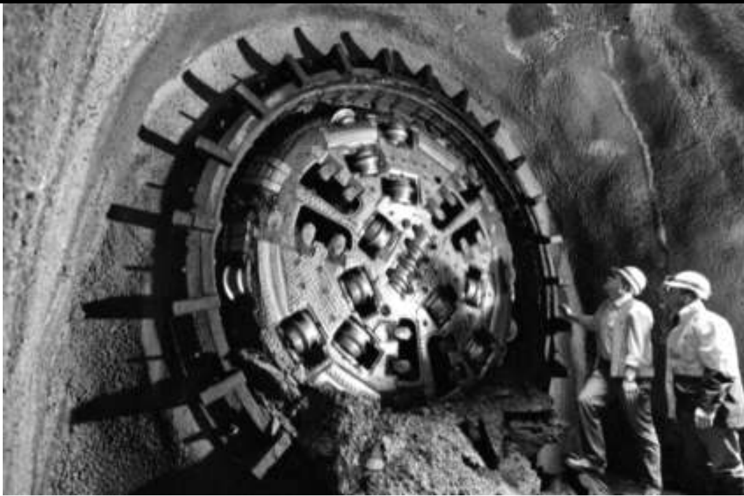
TBM "Victoria" breaks through at Carr St
