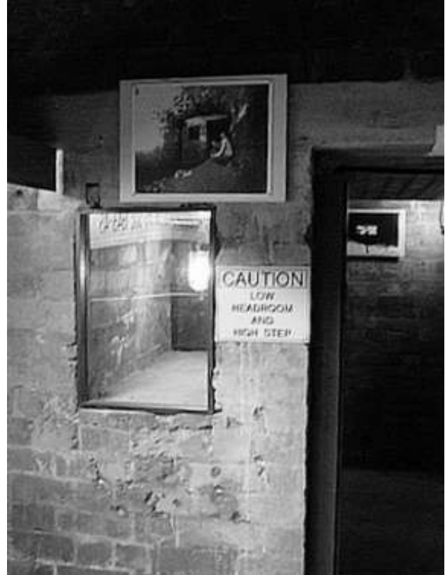
Bullet hole damage to walls. The tunnels were used by the SAS for live firing exercises in later years.
