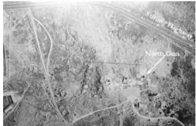
Aerial photo of the Leighton Battery site in 1947.
