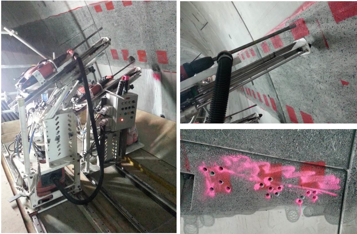
Figure 10 – CADS Production phase, reinforcement strikes
