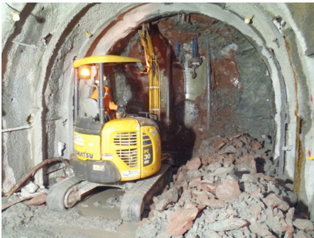
Figure 5 – Adit excavation and ground support
