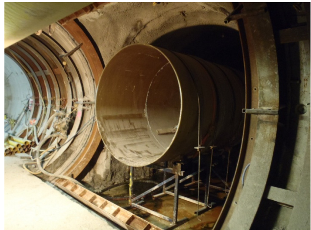
Figure 6 – GRP installed in adit
